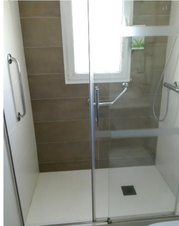
Replaced bath tubs for walk in showers in 2 studios
